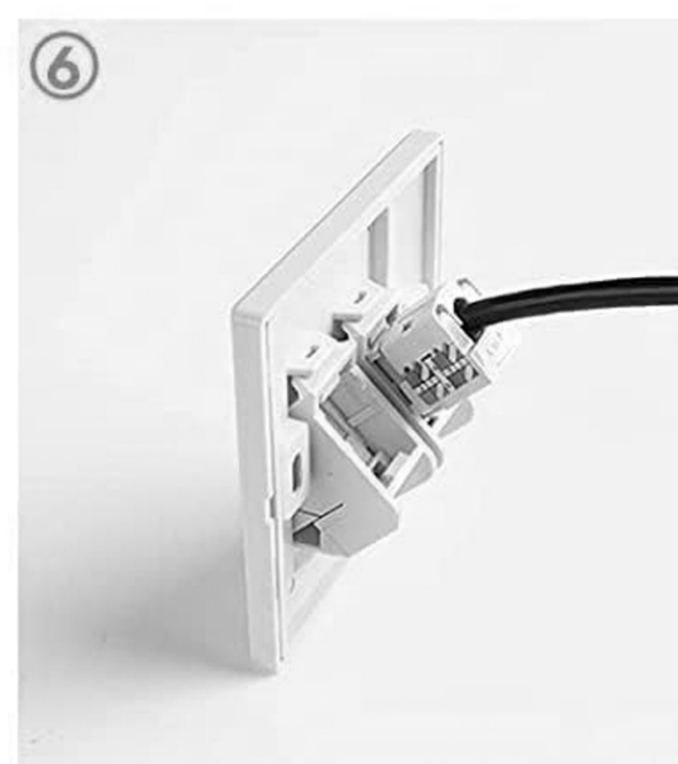
⑥ Insert the Keystone Wall Plate
